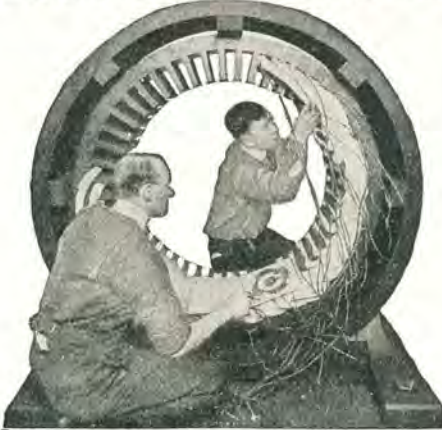
Student Winding a Stator
